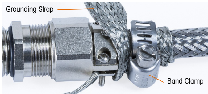
Figure 2-64: Ground Strap and Clamp Installed
